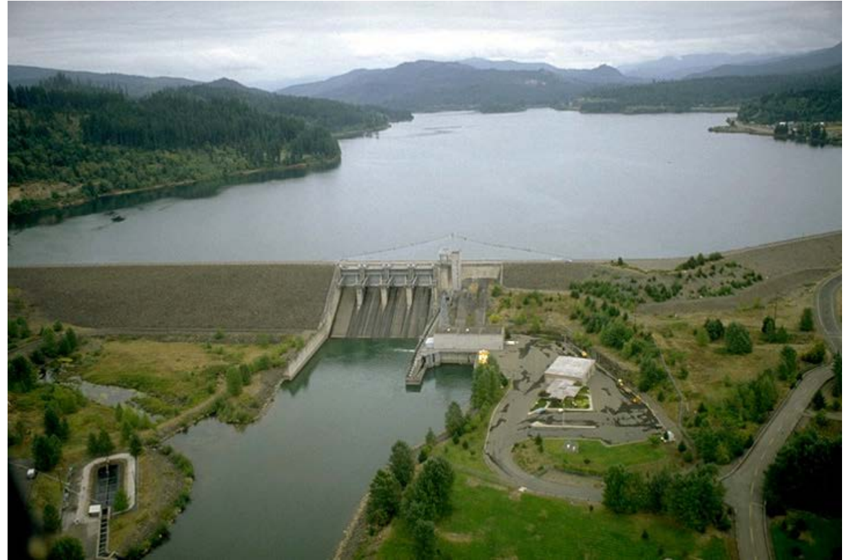
Foster Dam – USACE file photo
