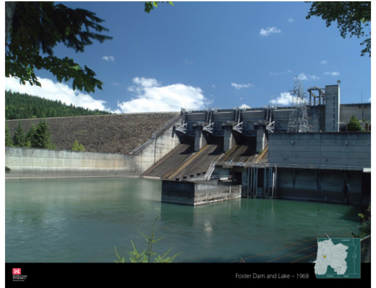
Foster Dam – USACE file photo
